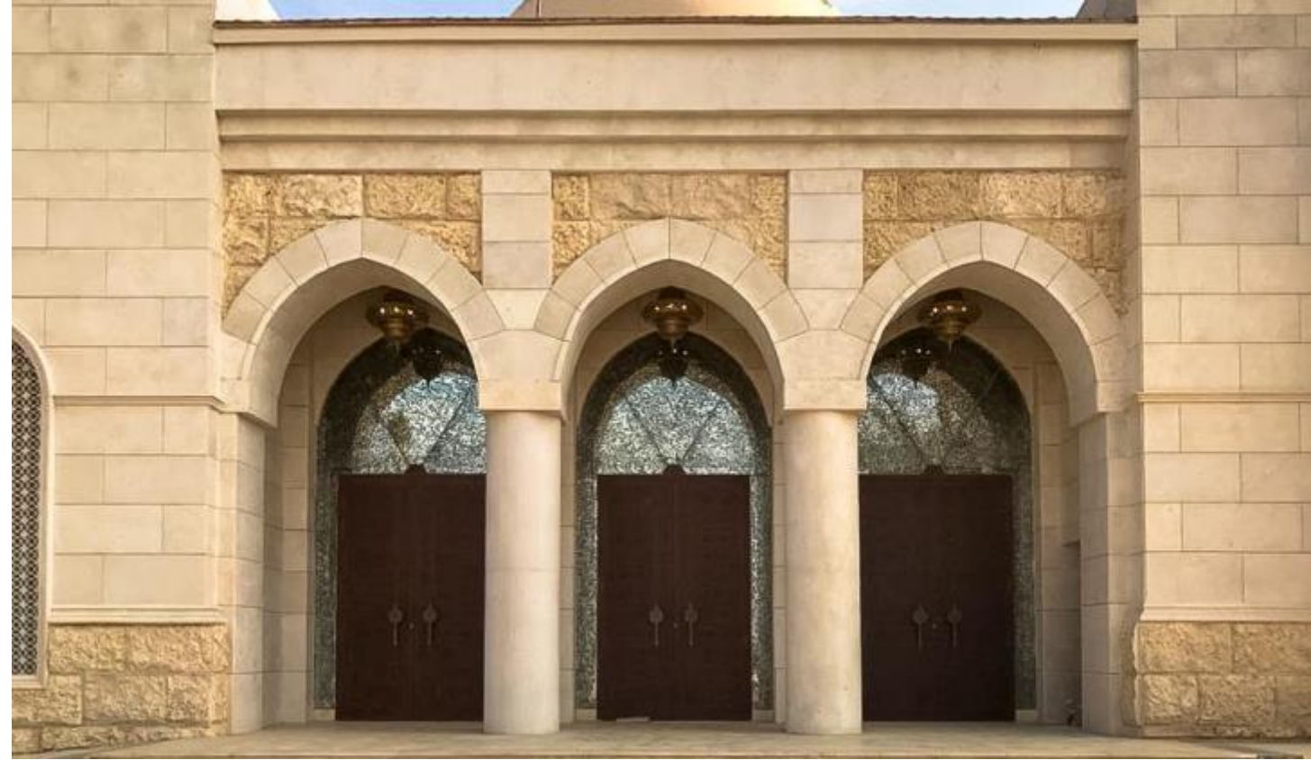
Main Mosque, Arts and Cultural Center, New Administrative Capital
